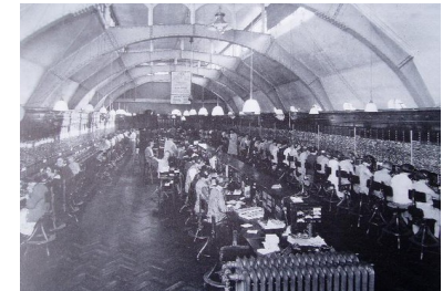
Telephone Central Office in London, 1926
