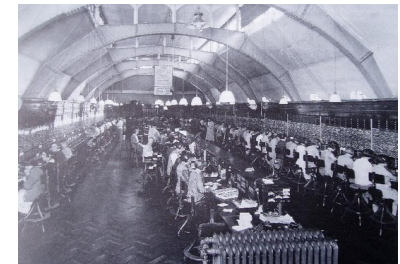
Telephone Central Office in London, 1926
